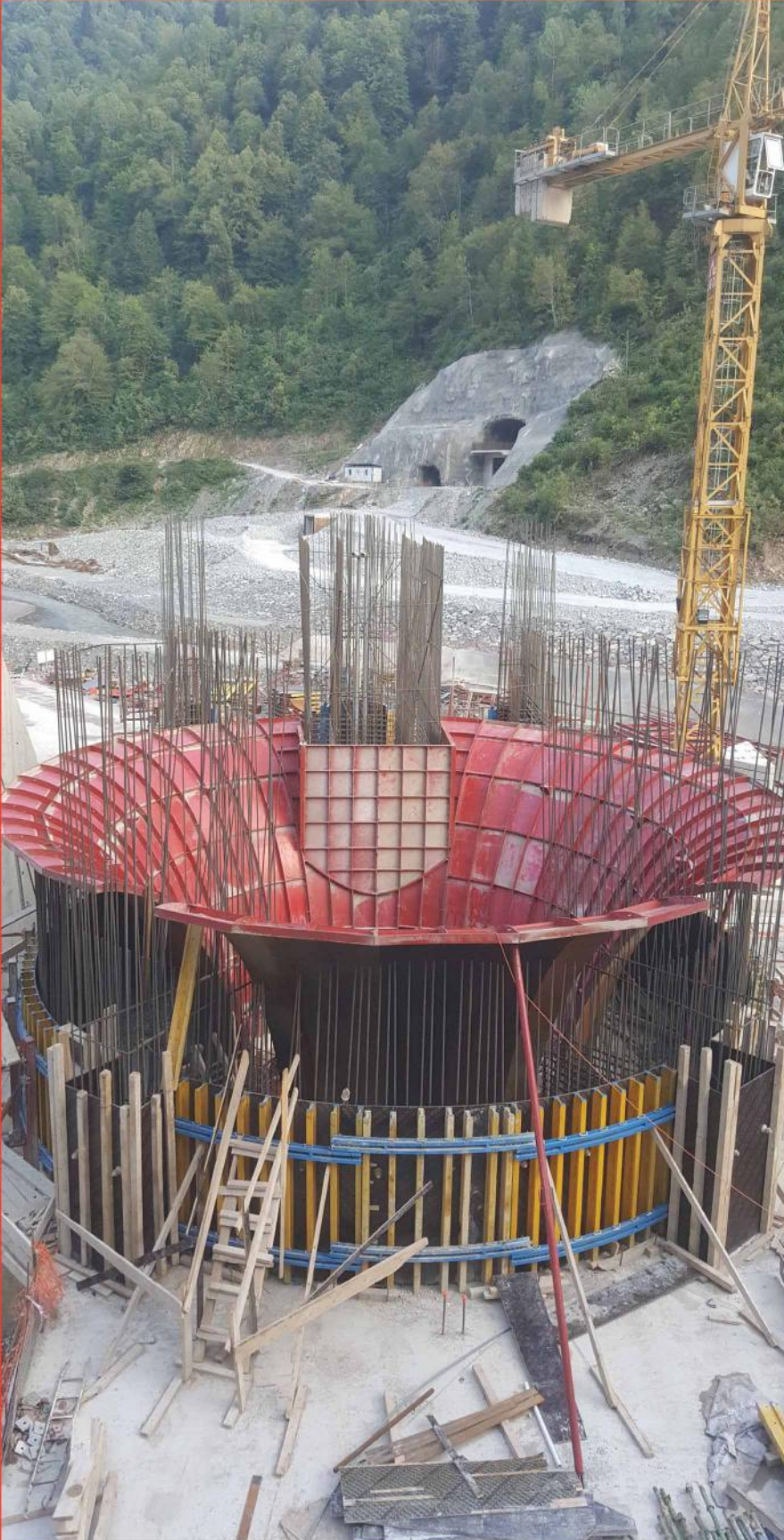
Pipette formwork and climbing formwork for a HES project, Turkey
