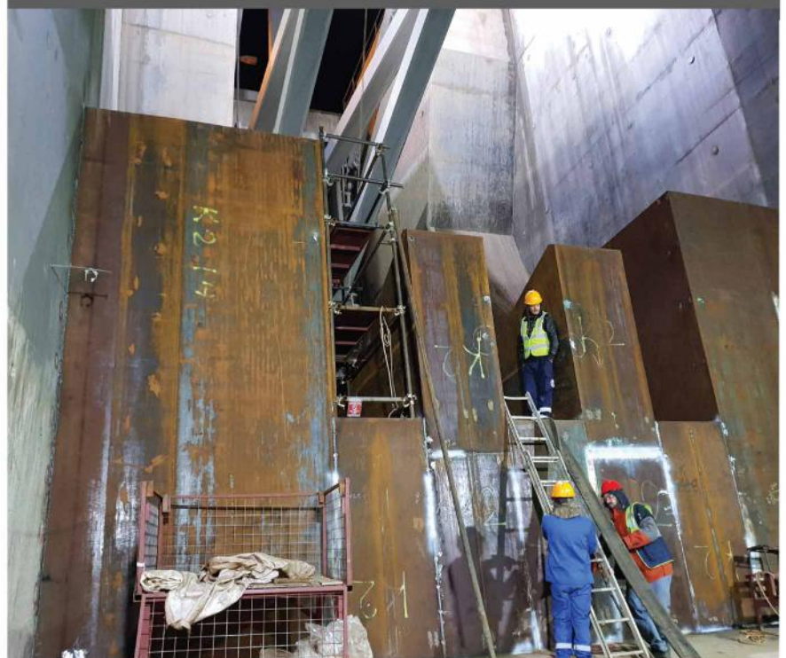
Mosul Dam Dentate Steel Construction
