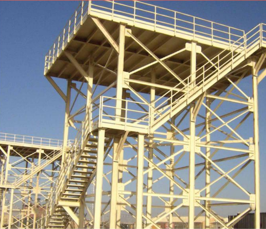
Communication Platform / Watchtower US Engineering Corps, Afghanistan
