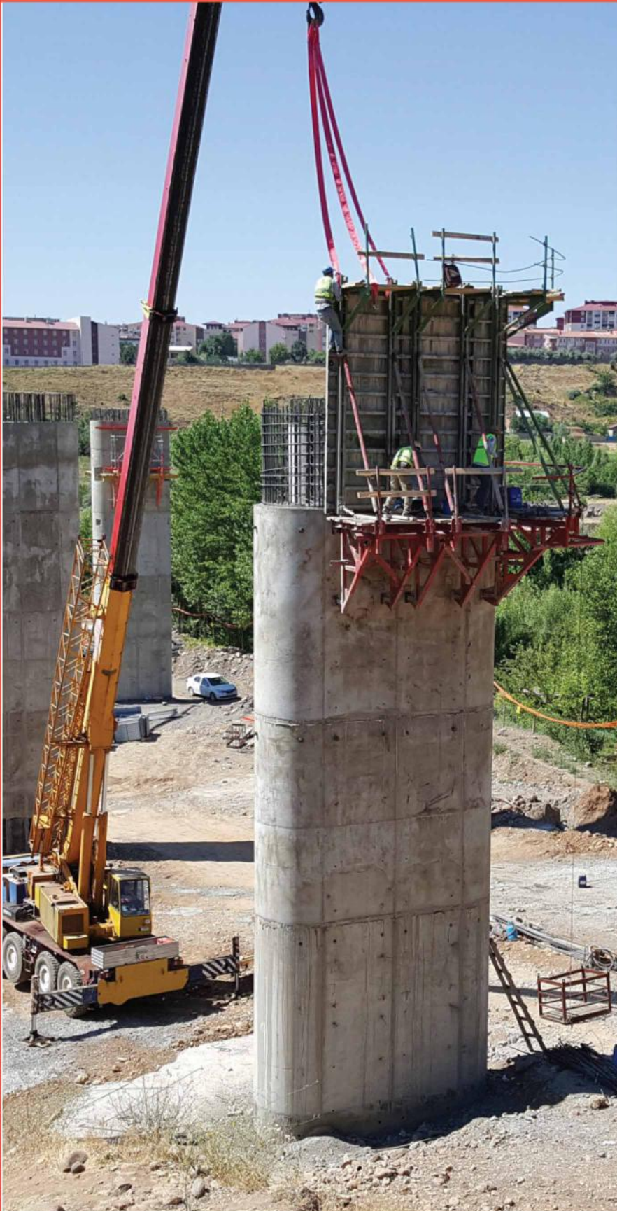
Bridge Footing Column Self Climbing Formwork
