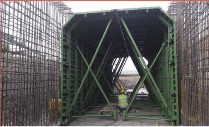
Box Culvert Formwork, Iraq
