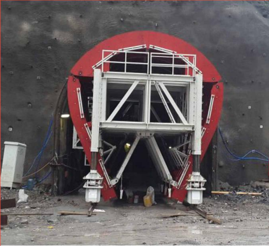
Tunnelling in Turkey
